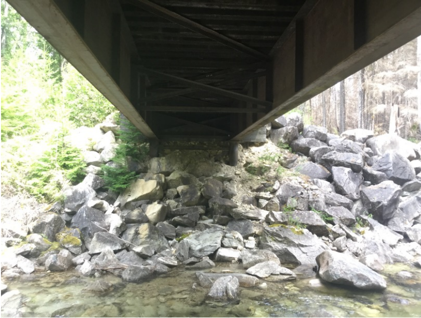
Right Bank Abutment
