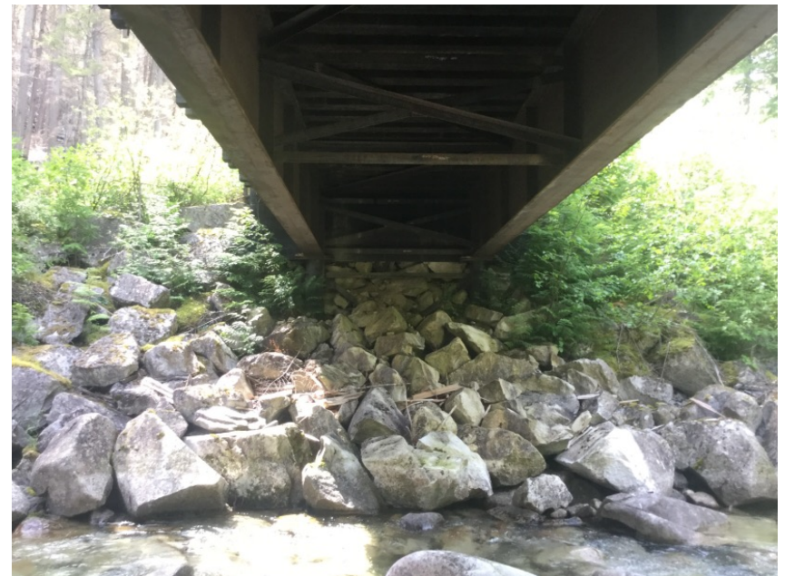
Left Bank Abutment
