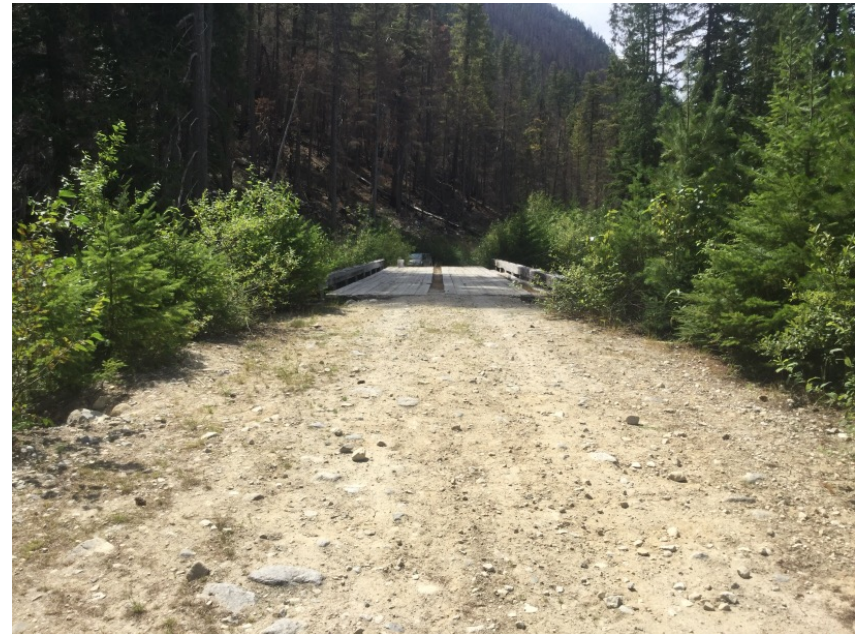
Right Approach Facing Bridge
