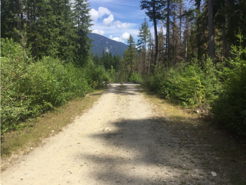
Left Approach Facing Bridge
