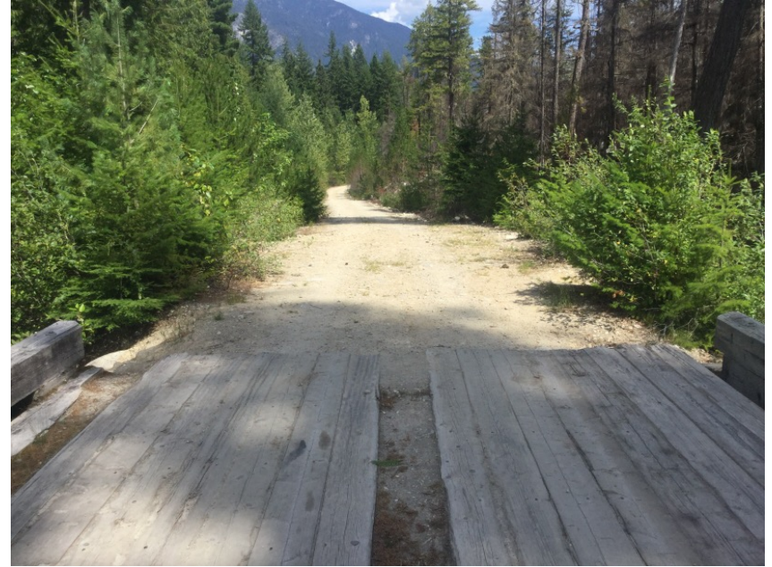
Right Approach Facing Away From Bridge
