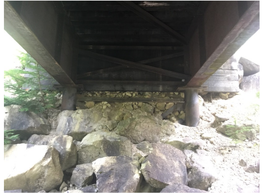
Right Bank Abutment
