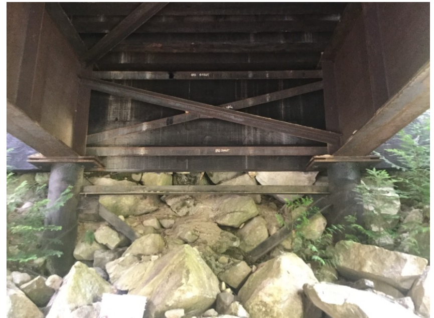
Left Bank Abutment
